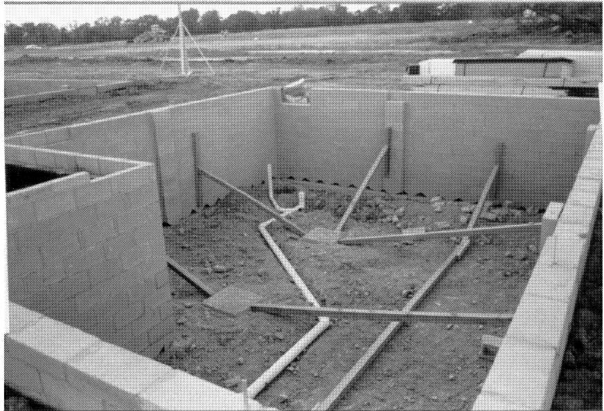
Figure 8-6: Bracing of Masonry Foundation
