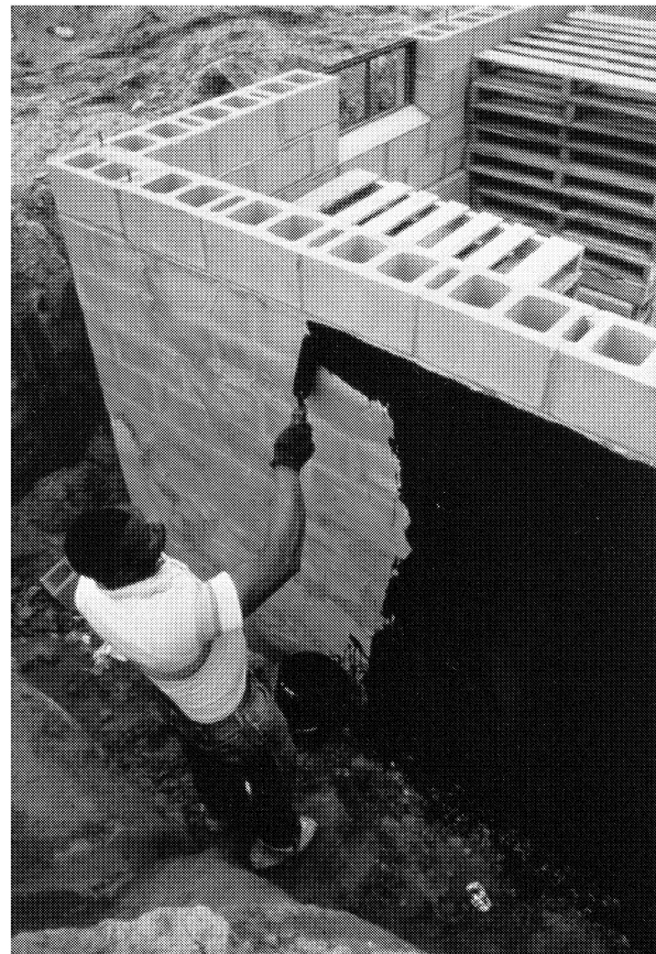
Figure 4-10: Applying Exterior Bituminous Sealant
